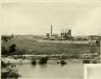
WEST END FURNACE
